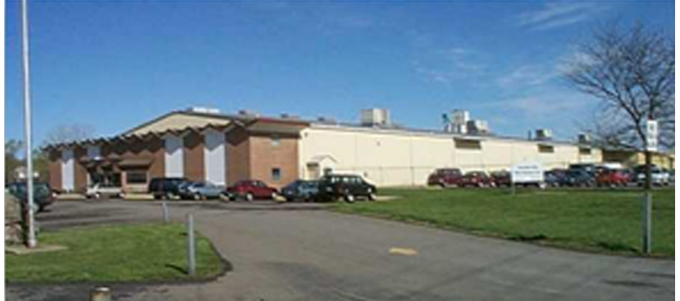
Junction City Wire Harness' 85,000-square-foot facility
